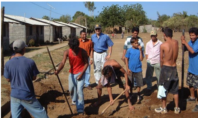
Execution of works: by involving the residents.
